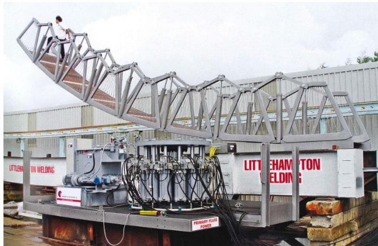
Rolling Bridge with exposed hydraulics
